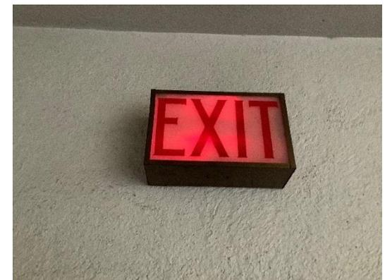
Photo E-6 – This exit sign in the RE Wing appears to have an LED light bar inside it. Exit signs in Metcalf Hall may still have incandescent lighting and replacement LEDs should be installed.
