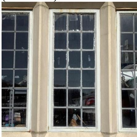
BE-18 -- This window in Metcalf Hall is the dominant window type: casement, single pane, leaded glass. Inefficient due to air infiltration and low R value.
