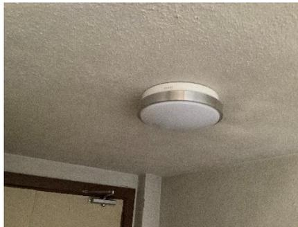
Photo E-5 – And LED surface-mount fixture in a hallway of the RE Wing.
