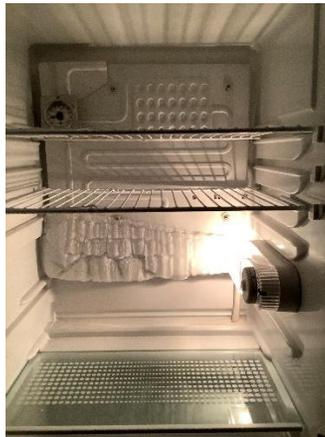
Photo E-11 – The small beverage fridge in the Symmes kitchenette was empty but set at such a low temperature that ice formed on the coils. Adjust to a warmer setting. Or turn it off until in-person events resume.
