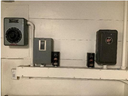
Photo E-7 – These lighting dimmers used to operate the Sanctuary lighting but were not replaced when lights were upgraded to LED, and are unlikely to be compatible.
