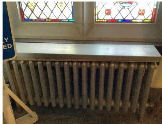
H-17 – Steam radiators, like this one in the Main Street entry, are the most common heat delivery system.
