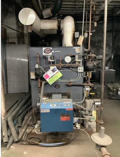
H1 — WUS has a large steam boiler that serves the entire building. Even if only 1 zone calls for heat the boiler must fire up so in a building with variable use patterns by zone, this is inefficient.
