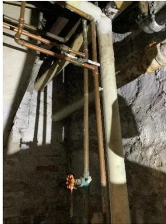
H-26 – The hot water pipes from the Ruud tank hot water heater are uninsulated, thus lose a lot of their heat on the long path to the Metcalf Kitchen and bathrooms. Insulating these pipes is a simple project with this insulation readily available at the hardware store or home center.
