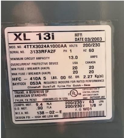
H-7 – The label for the office air conditioner shows the unit was manufactured in 2003, thus is nearing the end of its useful life.
