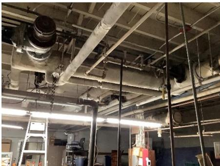
H-10 — Main steam pipe in boiler room with good insulation.
