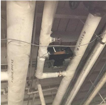
H-13 -- Pipes for Parish House (serves RE Wing, Metcalf and some uncontrolled areas) and Cloister (Offices) with controller for the Office zone.
