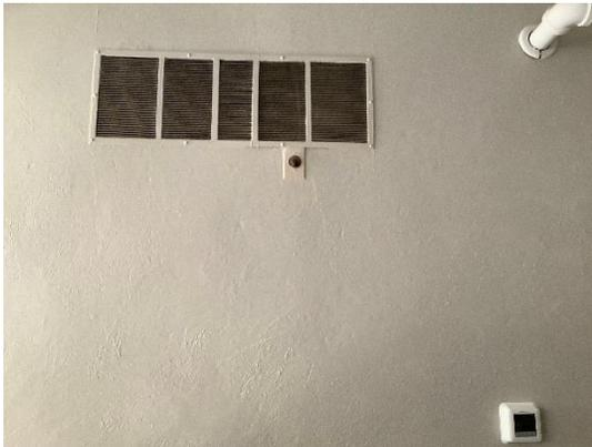
H-19 – This vent provides forced hot air to Winsor and should be used as the primary heat source. Thermostat at bottom right controls the blower.
