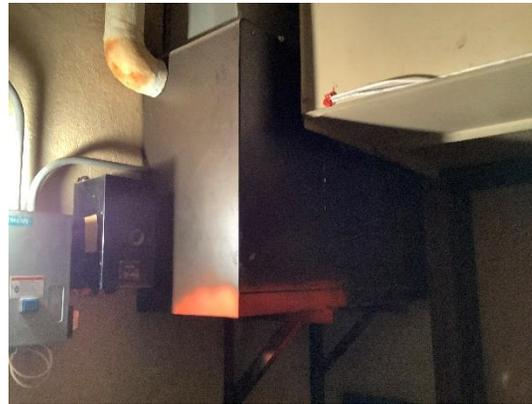
H-20– This blower unit in the closet off of Winsor delivers heat through the vent shown in photo H-15.
