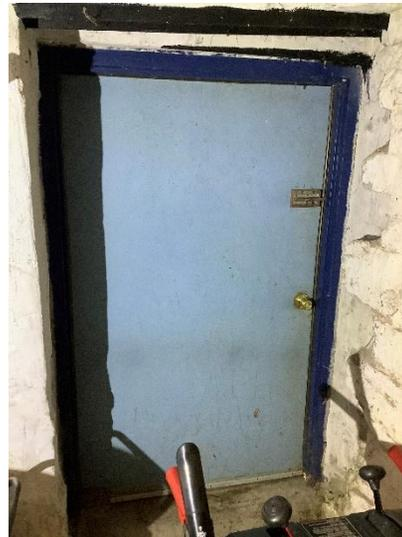
BE4 — Exterior door in the “snowblower room” needs weather stripping and 2-inch poly-iso rigid insulation applied. Water pipes in this room need a heat tape and these improvements may eliminate it.
