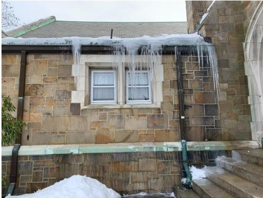
BE1 — Icicles and ice dams outside the accessible bathroom indicate little insulation in the roof.
