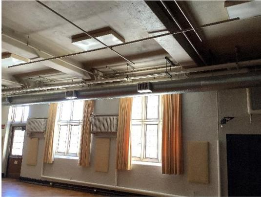
H-25 – The new duct work in Metcalf Hall (above the windows) connects to an ERV for dehumidification and fresh air in this space.
