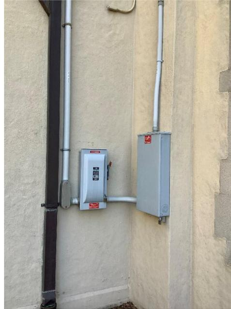
Photo E19 — The disconnect switch for the solar panels is located in the corner where the Metcalf Hall connects to the Office section
