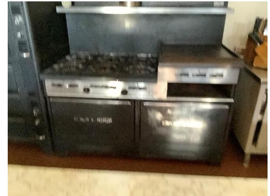
Photo E-16 -- The range in the Metcalf kitchen is old. MassSave incentives will help replace this with a modern, pilotless range. Or consider upgrading to electric induction.
