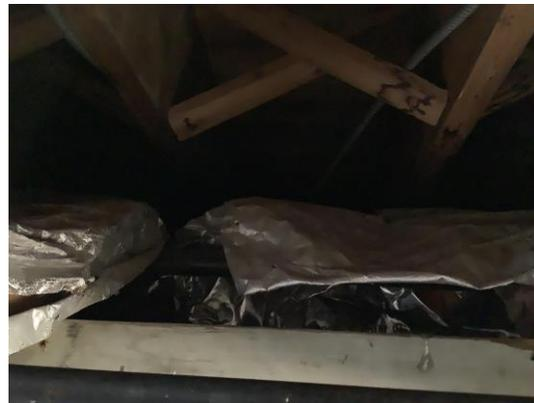
BE 15 -- Insulation in the ceiling of the RE Wing, viewed through a hatch in one of the classrooms. This is insufficient but could be supplemented with blown-in insulation.
