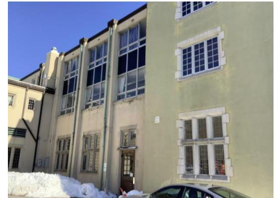
BE 17-- Exterior of the RE Wing. Large single pane windows with aluminum frames have poor thermal performance. The wall is stucco over cinderblock with no insulation.
