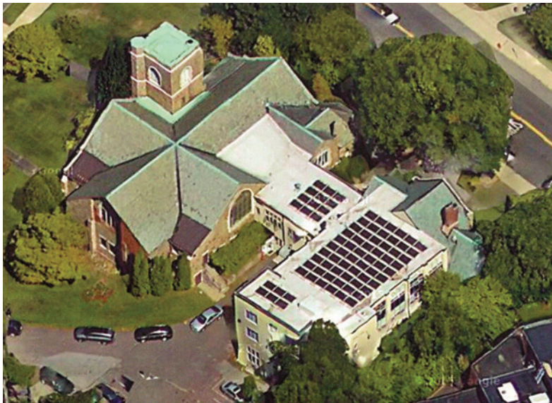
Solar Panel Array
